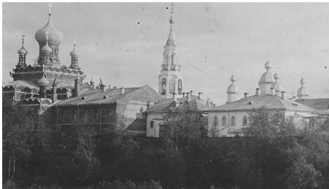
Fig. 1. The northern facade of the Sophia Monastery in Rybinsk, late 19th – early 20th century
